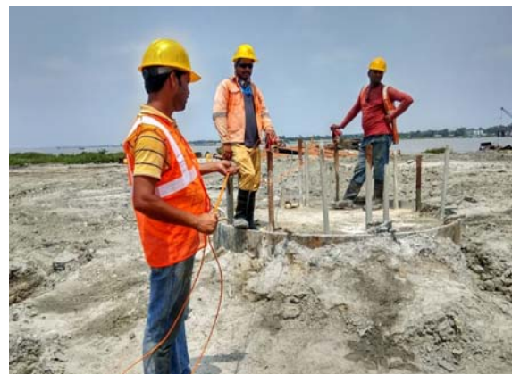
Fig. 10. Pipes cast in pile for CSL test
