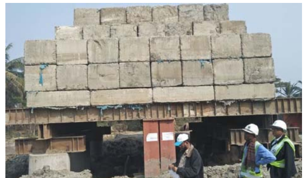
Fig. 5. Static pile load test in progress
