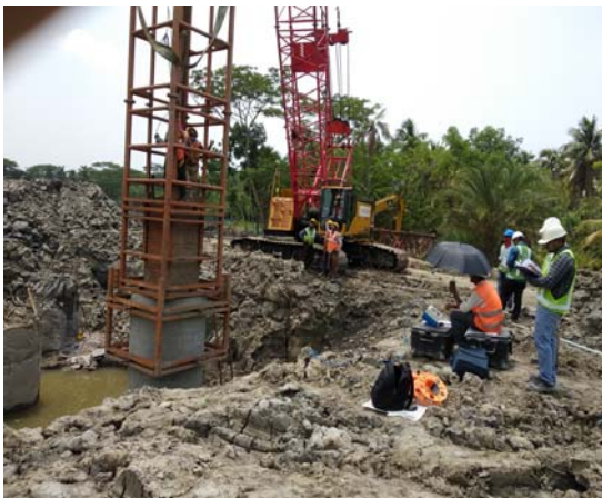
Fig. 6. HSDLT test in progress
